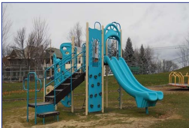
A work in progress, the new, improved Beekman Park playground on Peoples Avenue
